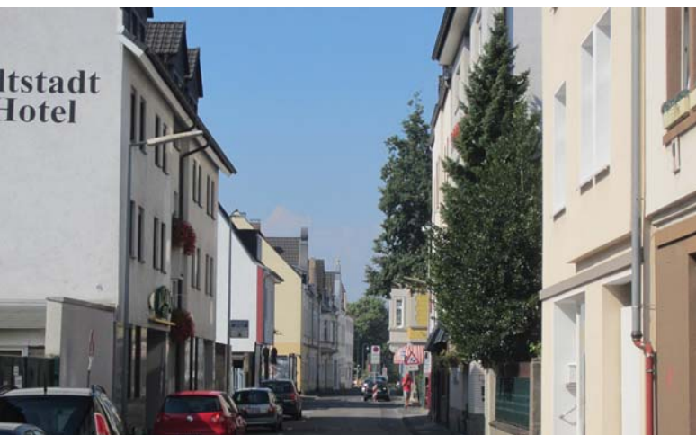
Altbausubstanz in Wiesdorf
